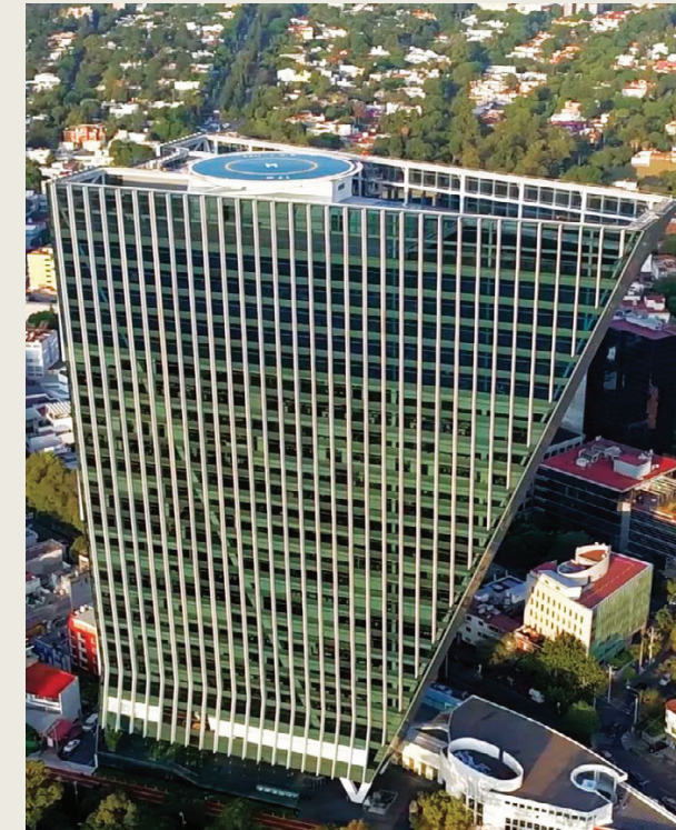
Torre Virreyes LEED Silver • Mexico City, Mexico • Commercial building • Product: Multi V Water II
