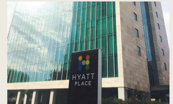
Hotel Hyatt Place LEED Certified • Santiago, Chile • Accommodation facilities • Product: Multi V Water Heat recovery
