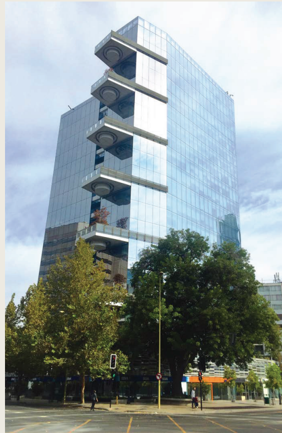
Territoria El Bosque LEED Certified • Santiago, Chile • Commercial building • Product: Multi V III Heat recovery
